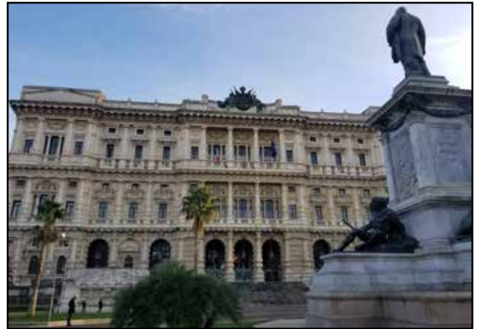
The Palace of Justice in Rome, Italy, is often called "il Palazzaccio" (the "bad palace") for its discordant architecture.
