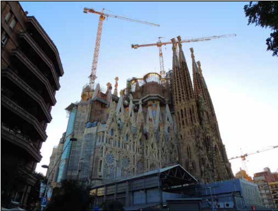
Construction continues on Basilica de la Sagrada Família in Barcelona, Spain.
