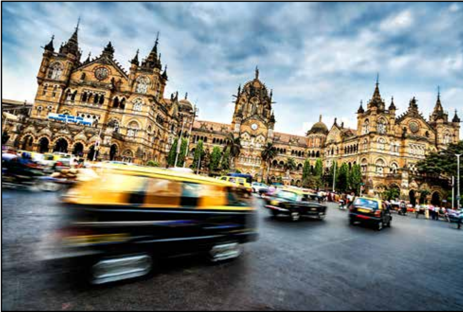
Chhatrapati Shivaji Maharaj Terminus (formerly Victoria Terminus), an iconic railway station in Mumbai, functions as the headquarters of the Central Railway. Photo: iStock.com
