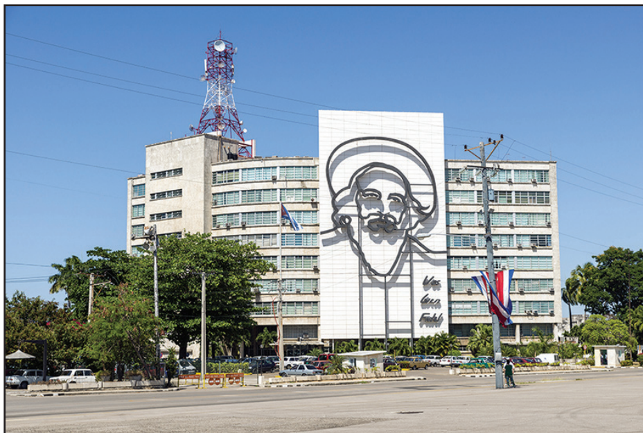
A steel outline of Camilo Cienfuegos' face adorns the Ministry of Informatics and Communications building at the Plaza de la Revolución in Havana. (Villorojo/Shutterstock.com)
