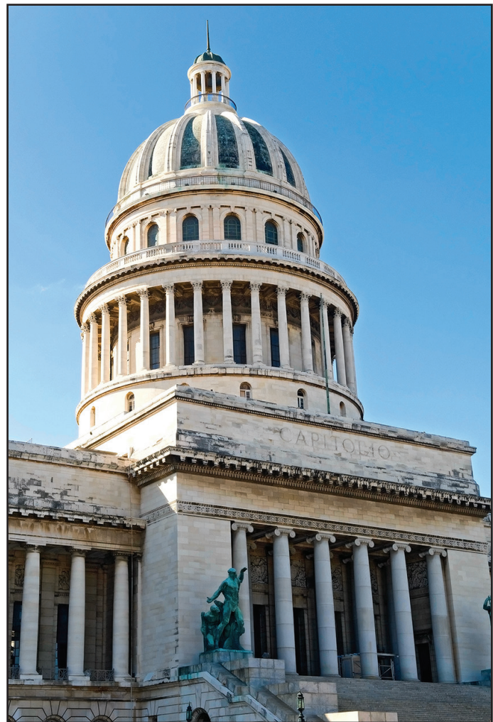
This building houses the Cuban Legislature. Since 1976, the Cuban Legislature has structured the principle of independence of the government and Cuban companies. (Krechet/Shutterstock.com)
