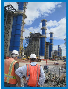
The Caribbean’s largest power plant under construction in Trinidad and Tobago
